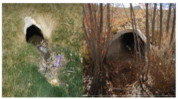
Require sediment removal when Sediment depth is 6-12 inches
